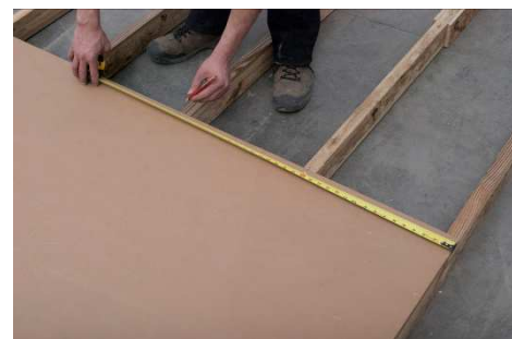
(32) Before you finish attaching the first row flooring to the joist, make marks 12" on center for a guide to adjust the joist when nailing. Then finish nailing the first row flooring.
