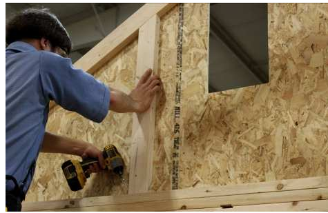
(129) Fasten the bottom of the gable brace on both sides.
