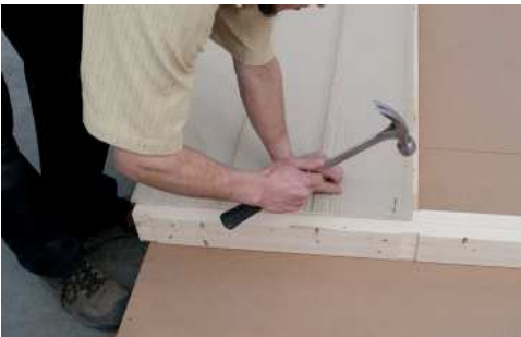
(47) Nail along the top, after making sure the siding is flush with the center of the double top plate as shown. Use an 8" to 12" nail spacing.
