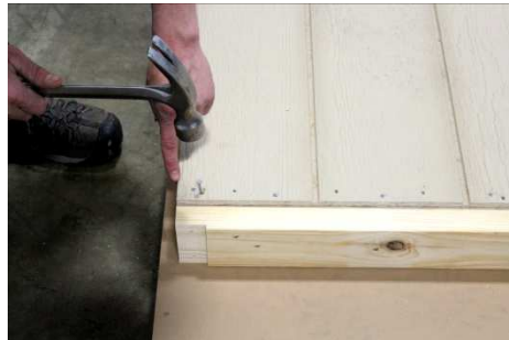
(45) Starting with the left piece, place the siding even with the center of the double top plate, and flush with the wall stud.
