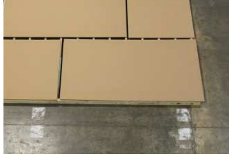
(26) Start on the front right corner with a full 4'x8' piece, making sure flooring is flush with floor joists.
