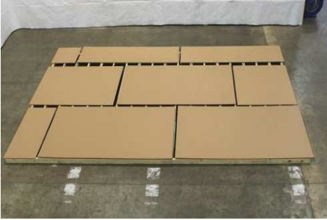
(25) Layout the flooring as shown.
