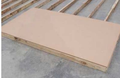
(29) Nail along the front side, again; making sure flooring is flush with the band board.
