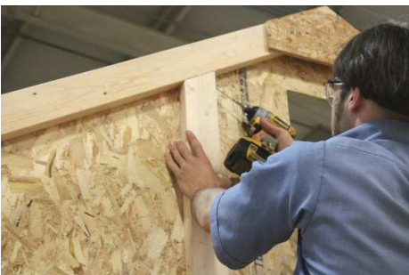
(128) Locate the 4 gable braces then fasten them at the siding splices in the peak, using 3" screws.
