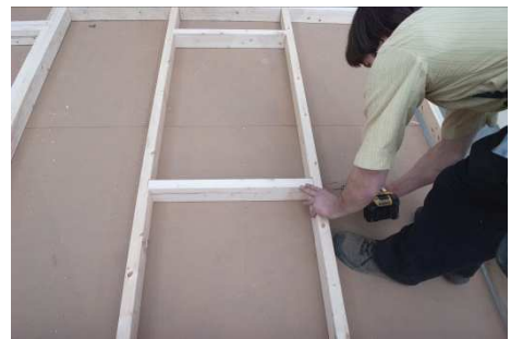
(76) Fasten window studs with dados, to the window blocks, using two 3” screws.
