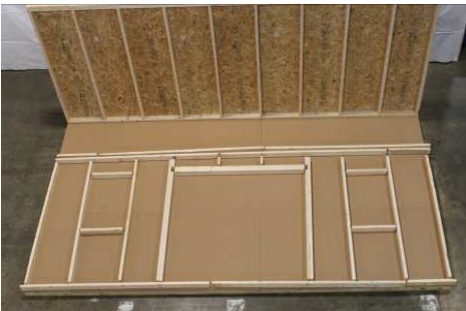
(74) Locate and lay out the parts to assemble the front wall.
