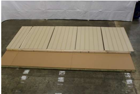
(44) Lay out siding as shown here, with the overlap towards the left.
