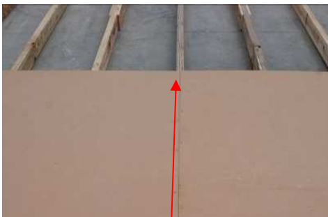
(31) Center the floor joist evenly with the flooring splice, then nail the corner, after making sure flooring is tight against, and flush with the previous piece. Nail this piece, using the same methods as the previous piece.
