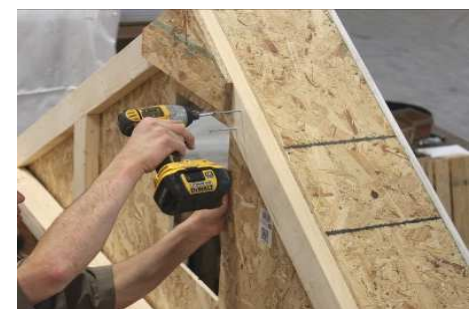
(127) Properly secure gable overhangs with 3" screws, every 10 to 12 inches.
