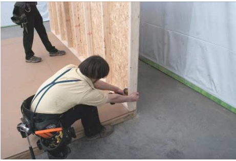
(68) Fasten to floor, using two 3” screws at every stud, trying to hit the floor joists.
