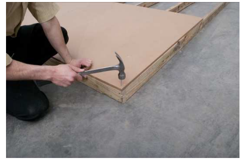
(27) Attach the corner of the flooring, using 2" nails.
