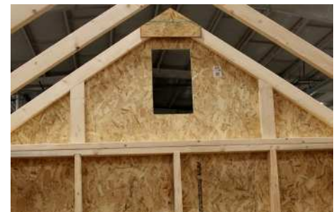
(130) Fasten the other gable brace on this gable, then repeat for opposite gable. Next, fasten the siding splices to the gable braces on the outside.
