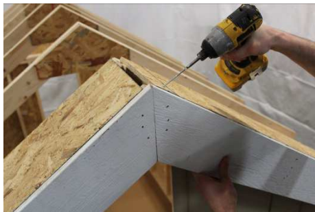
(125) Correct! Fasten firmly, using a 3" screw.
