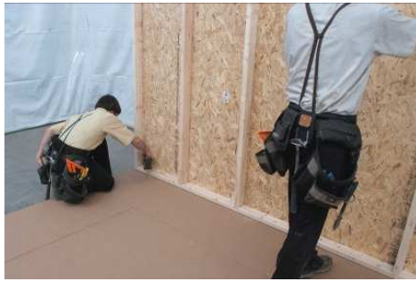
(69) Repeat for the rest of the wall, again; making sure wall is in against the floor frame.
