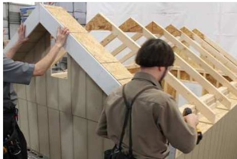
(123) Install right gable overhang, repeating previous steps.
