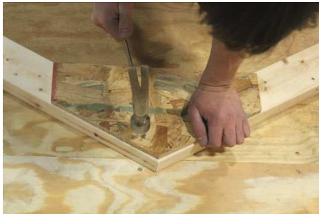
(119) Assemble each rafter by attaching one gusset to each side of the rafters as shown, using a total of ten 2" nails per gusset.
