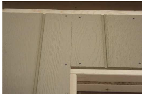
(78) Fasten the siding pieces above the doors, and keep it 3/4" above door header as shown; before nailing.
