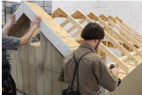
(135) Install right gable overhang, repeating previous steps.
