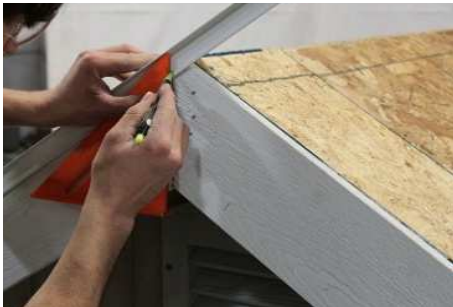
(209) Make a mark on the drip edge, parallel with the gable splice.
