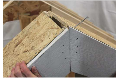
(136) Incorrect! Before fastening the overhangs on the top, make sure the splice is uniform, as shown in next step.
