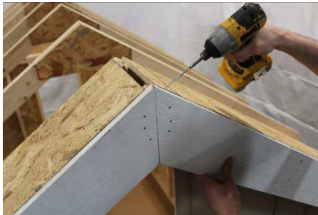
(137) Correct! Fasten firmly, using a 3" screw.
