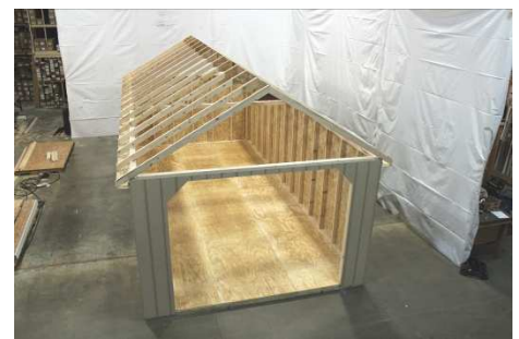
(124) Install the rest of the rafters, 24" on center, or in every dado groove on the top plate. Repeat, till all rafters are installed.
