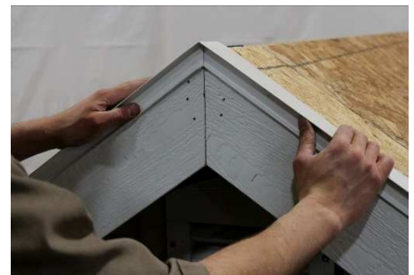
(211) Bend around the top as shown. This top piece should overlap the bottom piece. Do not fasten it till the bottom piece is installed on the other side. Finish installing the rest of the drip edge.
