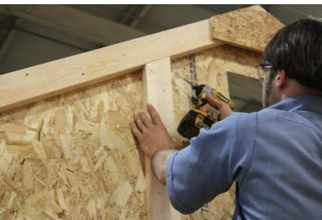
(140) Locate the 4 gable braces then fasten them at the siding splices in the peak, using 3" screws.
