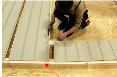
(75) Starting with the piece beside the door, place the siding even with the center of the double top plate, then make sure siding has 3/4" reveal along edge of door frame, before nailing.
