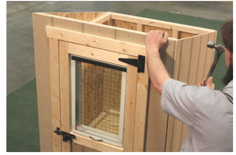
(31) Fasten wall securely before moving to next step.
