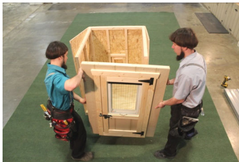
(30) Insert the front wall in between the left and right wall, then fasten the bottom, as well as both corners, as done in previous steps.
