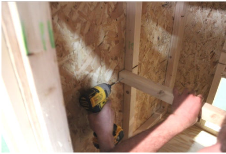
(41) Fasten opposite side of roosting bar, again using (1) 3" screw.
