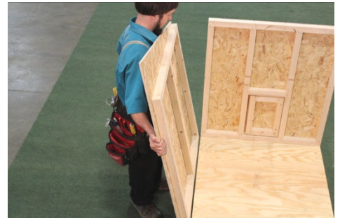
(25) Locate and position the left wall section, making sure you have the correct wall. Low end should align with the back wall. See example!
