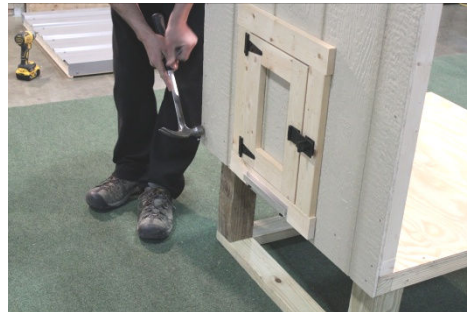
(24) Once the wall is placed correctly, fasten it to the floor as shown, using a total of (4) 2" siding nails.
