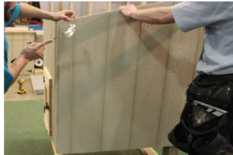
(27) Now, fasten the corner of the wall, using (3) 2" nails, and making sure the corner framing is flush with back wall.
