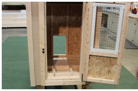
(42) Locate the (3) laying boxes, & place them in the position of your choice. Nesting Box Position #1
