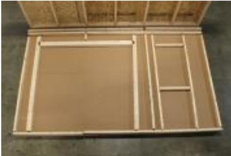
(56) Locate and lay out the parts to assemble the front wall.
