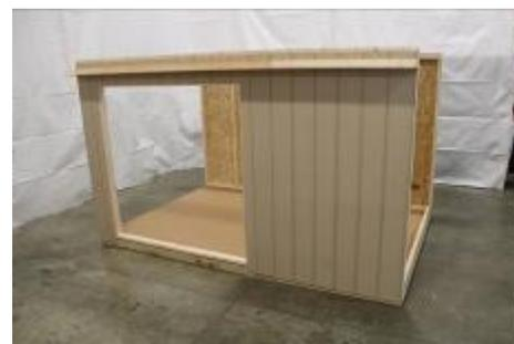
(69) Set the front wall, again: making sure edges of wall are flush with edges of floor. **It is VERY important that a person holds the wall in place until wall is attached firmly to floor, or braced.**
