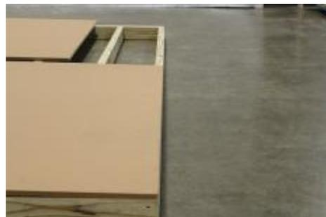
**(16)** Nail along the gable, again; making sure flooring is flush with the floor joist. Use an 8" to 12" nail spacing.
