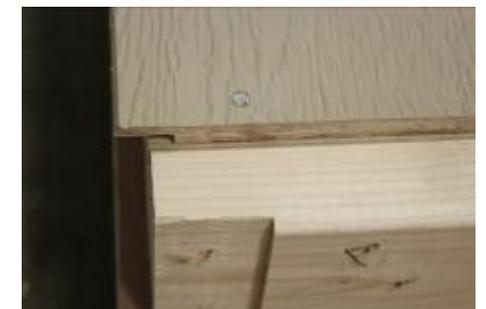
**(34)** Nail this corner with one 2” nail, before moving to the next step.
