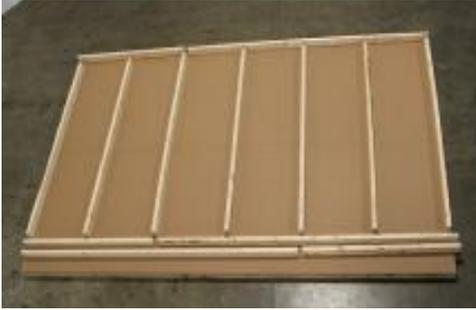
**(26)** Be sure to alternate top wall plate splices.
