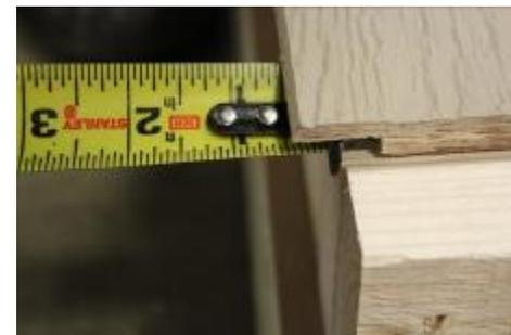
**(33)** Place the siding even with the center of the double top plate, and 1/2” out over the wall stud.
