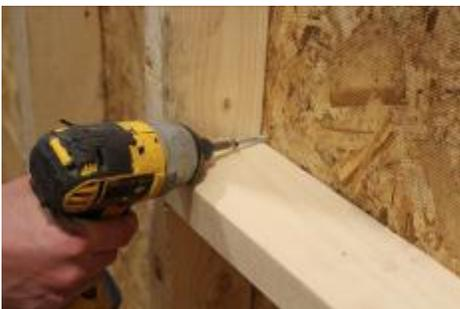
**(86)** Run a 2" screw through siding at each corner of the window.
