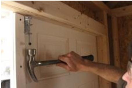
**(155)** Pull door in, tight against the frame, then make a mark for the inside latch pin. Repeat on the bottom.
