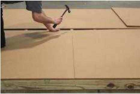
**(19)** Center the floor joist evenly with the flooring splice, then nail the back right corner, after making sure flooring is tight against, and flush with the previous piece.
