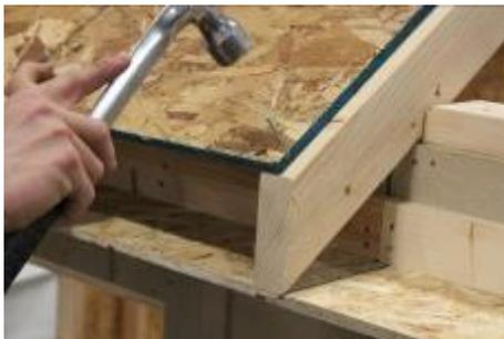
(119) Make sure sheathing is centered on rafter, then attach at bottom right corner. **Important! Nail along the bottom at every rafter, before moving to next step.**
