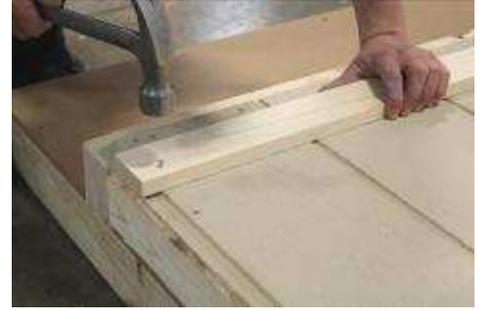
(46) Align bottom of 1x3 soffit strip with chalk line, and keep flush with wall frame, then secure, using 2" nails, and nailing on every stud.
