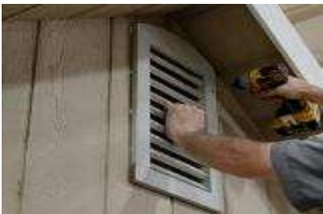
**(140)** Install the vent, making sure it is straight, then fasten, using two 1-1/4" screws per side. Repeat for the other vent on opposite gable.
