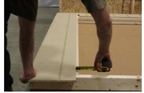
(64) Make sure siding has 3/4" reveal along edge of door frame. then nail along door frame. Finish nailing this piece.
