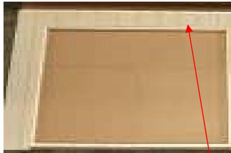
(66) Repeat with the next piece, making sure the siding has a 3/4" reveal on the top of door, as done in previous step.
