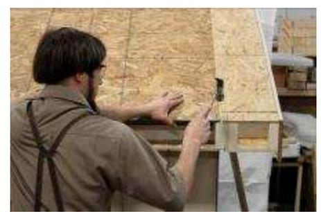
(121) Fasten the sheathing on the bottom right corner, making sure it is flush with bottom edge of gable rafter. **Important! Nail along the bottom, at every rafter before moving to next step!**
