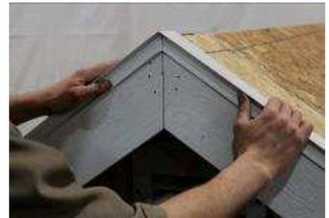
(175) Bend around the top as shown. This top piece should overlap the bottom piece. Do not fasten it till the bottom piece is installed on the other side. Finish installing the rest of the drip edge.
