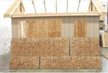
(116) Locate the roof sheathing, and scatter out as shown.
