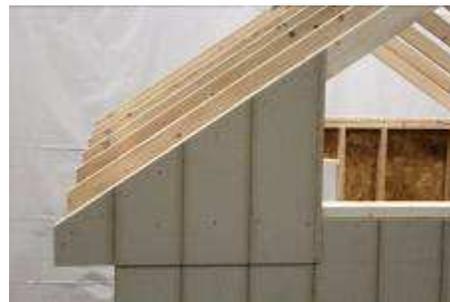
(102) **Correct!** Fasten firmly with 2" siding nails.
