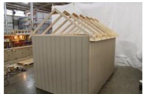
(97) Install the rest of the rafters, 24" on center, or in every dado groove on the top plate. Repeat, till all rafters are installed.
