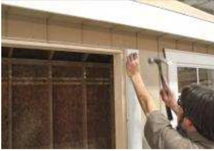
**(143)** Align trim flush with edge of siding and attach, using two - 2" trim nails spaced every 12 to 14 inches.
