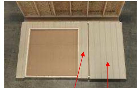
(67) Fasten the piece on the right side of door, using the same steps as the left side of door. Before fastening the last piece, check if the door opening is square. **IF NOT, pull the bottom of the wall left or right to adjust it, then fasten the last piece.**
