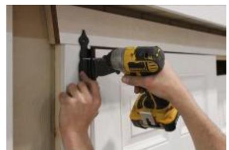
**(151)** Start with the left door, and fasten to trim using 2-1/2" black screws, and making sure you keep the top of the door down from the trim, approximately 1/4".
