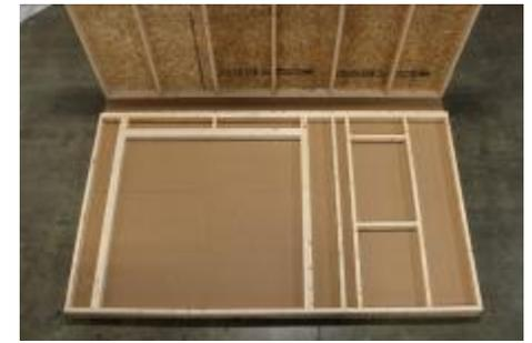
(61) Fasten the other studs, using the same pattern as the back wall.
