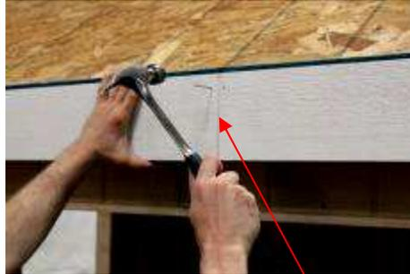
(129) Repeat previous steps, **making sure this piece is tight against the other piece as shown, before cutting to length and fastening.**
