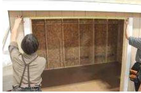
**(144)** Repeat for the other side, making sure the trim to trim opening is 72" before nailing. Check the measurement on the middle and bottom as well.
