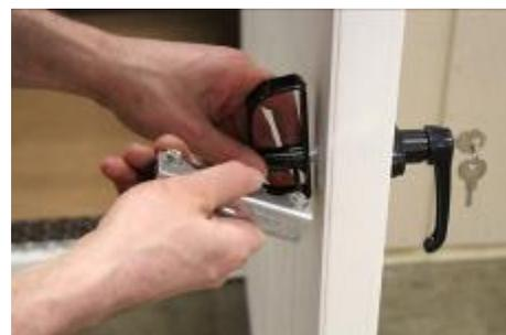
**(159)** Attach L-handle as shown using a 5/32 Allen Wrench. Adjust as needed.
