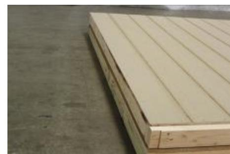
(42) Snap a line, even with the edge of the wall frame, then move to next step.
