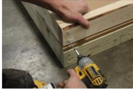
**(27)** Insert two 3” screws through the pre-drilled holes to attach bottom plate to each wall stud. Make sure bottom plate and wall studs are flush.
