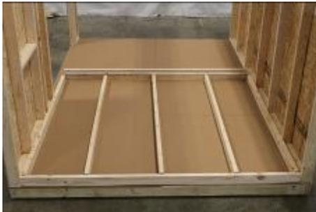
**(74)** Locate and lay out the parts to assemble the gable wall.
