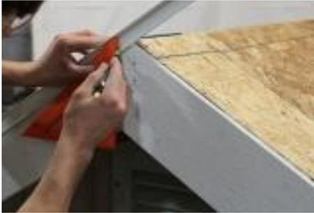
(173) Make a mark on the drip edge, parallel with the gable splice.
