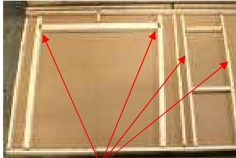
(57) Front wall is done much the same as the back wall except for the door and window studs. Locate double studs with dado for the door, and single studs with dado for the windows.
