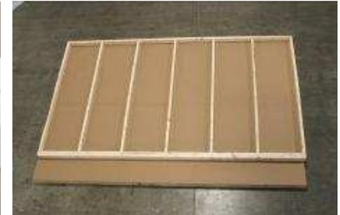
**(31)** Attach top plate, using 3” screws.
