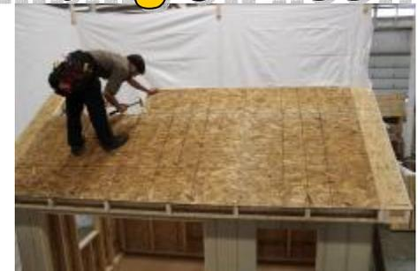
(124) Lay out the top row sheathing, making sure the splices are alternated, as shown in step (116) Fasten the last row securely, using the previous steps.
