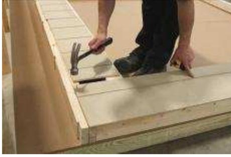
(63) Place the siding even with the center of the double top plate, then move to next step.
