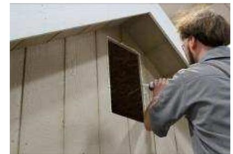
**(139)** Install vents, caulking around the perimeter, before installing.
