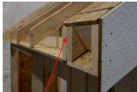
(105) Make sure the gable overhang is flush with the rafter, and tight in against the gable siding, as shown.
