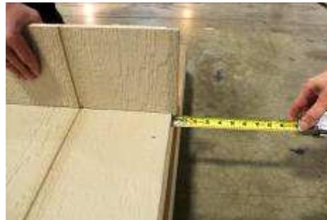
(48) Install soffit, starting on the right side of the wall, with the overlap edge sticking out 1/2" past the wall frame.
