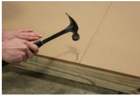
**(20)** Nail front right corner as shown, making sure the flooring is tight against previous piece, then nail along the splice.
