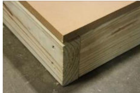
**(14)** Start on the front corner with a full 4'x8' piece, making sure flooring is flush with floor joists.
