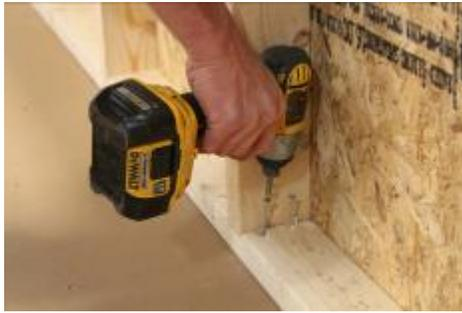
(54) Repeat for the rest of the wall, again; making sure wall is in against the floor frame.
