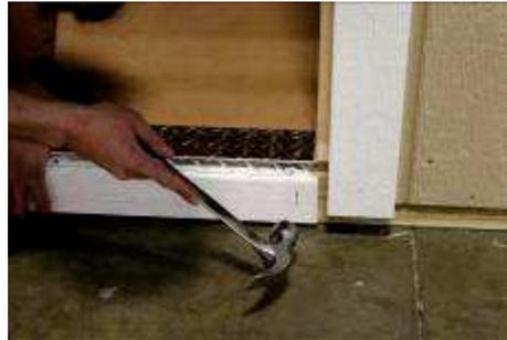
**(147)** Nail poly strip just below the diamond plate, using 2" trim nails and dividing it out evenly from left to right, ect.
