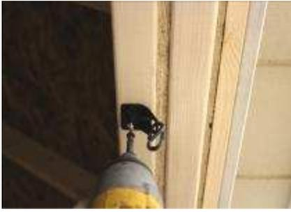
(161) Install the door spring fastener, using two 1-1/4" black screws.
