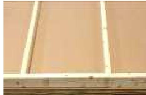
**(75)** Attach all wall studs to top and bottom wall plate.
