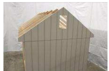
(103) Repeat with the rest of the peak pieces, making sure the bottom is flush with the chalk line.
