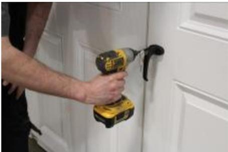
**(158)** Install latch using 2" black screws.
