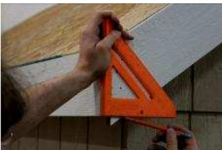
(131) Make a mark, flush with the fascia on the bottom as shown, then refer to next step.
