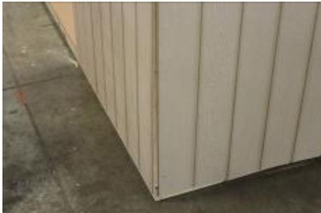
**(83) Incorrect!** Ensure bottom corner of siding is properly aligned.
