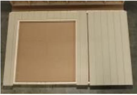
(62) Lay out siding as shown here, starting with the under lap towards the right.
