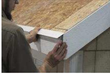
(171) Keep drip edge flush with the gable as shown, then nail every 12 to 14 inches, using roofing nails. (Nails not included.) Repeat for the next piece, keeping flush with the other gable.
