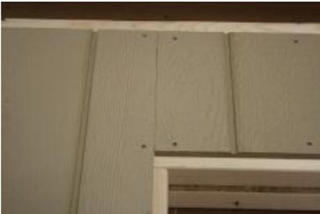
(65) Place the cut piece against the previous piece, and keep it 3/4" above door header as shown; before nailing.
