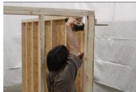
**(78)** Align gable wall framing flush with back wall framing and attach using 3” screws, every 8 to 12 inches. Repeat the process on opposite end.
