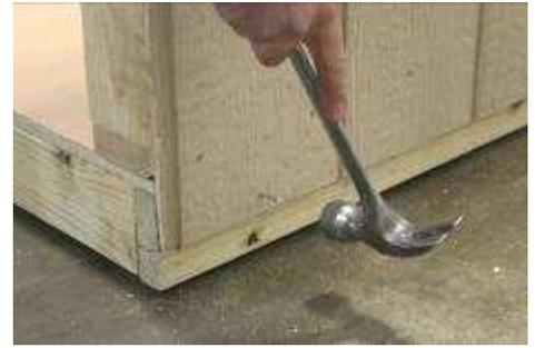
(55) Attach bottom edge of siding to floor, using an 8” to 12” nail spacing. **Do not leave the back wall standing alone for a long period of time, without firmly bracing it.**
