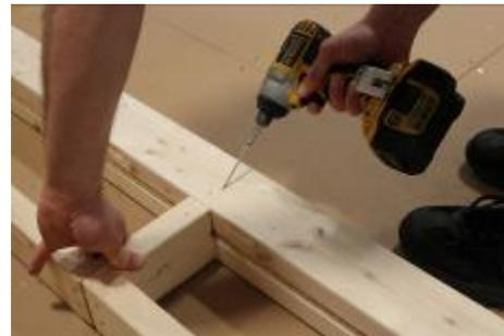
(60) Toe screw door header to door blocks, as shown.
