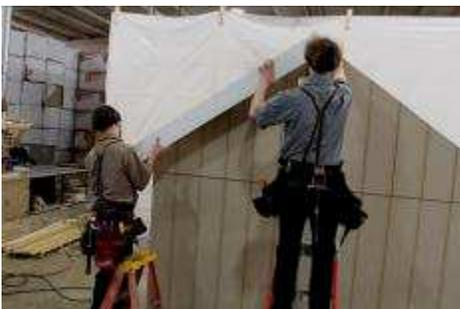
(104) Starting with the left gable overhang, put the overhang in place, then refer to the next step before fastening.
