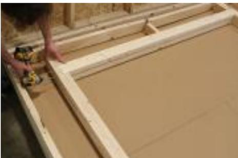
(59) Fasten door studs with dados, to the door header, using four 3” screws.
