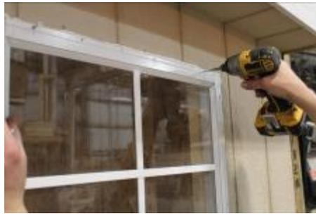
**(135)** Install window, making sure it is straight, then fasten it, using three 2" screws per side.
