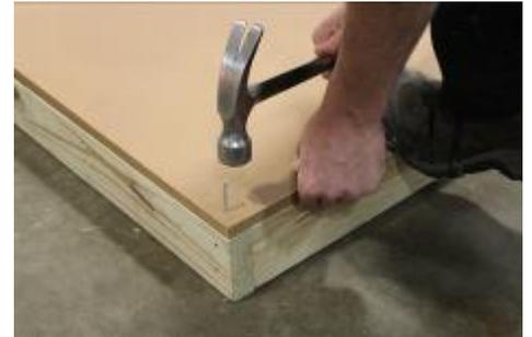
**(15)** Attach the corner of the flooring, using 2" nails.
