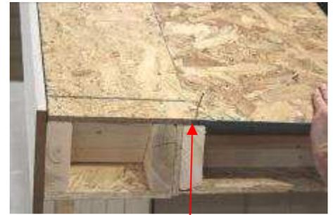
(118) Starting with the left piece, push roof sheathing tight against the gable overhang, and align flush with bottom edge of gable rafter, then attach, using a 2” nail.
