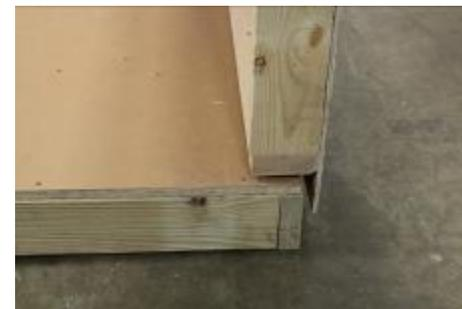
(51) **INCORRECT!** Wall needs to be flush, and in against the floor frame, and down against the flooring.
