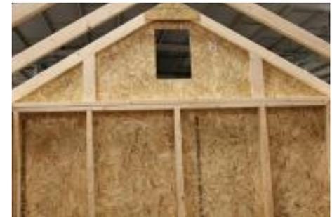
**(115)** Fasten the other gable brace on this gable, then repeat for opposite. Next, fasten the siding splices to the gable braces on the outside.
