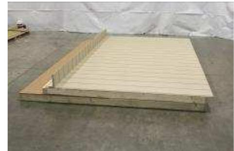
(49) Fasten the rest of the soffit much the same way as the siding. Last soffit piece should overhang by 1/2" as well. If necessary, cut to fit.
