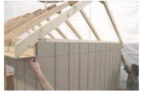
(100) Snap a chalk line 1/4" below the bottom of the soffit as shown.
