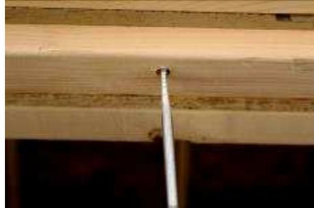
**(156)** Drill a hole, with 5/16" drill bit, using the pre-made marks.
