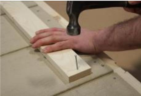
(47) Repeat for the rest of the soffit strips, making sure the bottom of soffit strip is even with the line.
