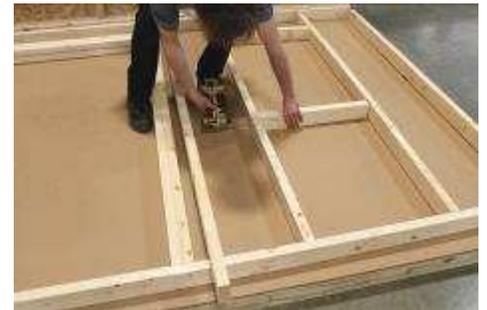
(58) Fasten window studs with dados, to the window blocks, using two 3” screws.
