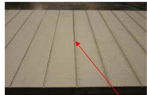
(40) Nail along the splice, making sure the splice is parallel, and looks similar to the other grooves.
