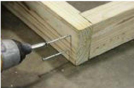
(7) Begin with the end joist, making sure the band board is flush with the joist.
