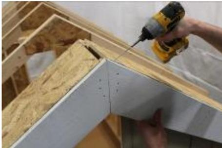
**(110) Correct!** Fasten firmly, using a 3" screw.
