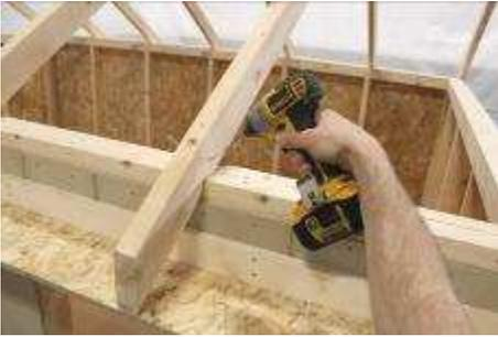
(98) Toe screw all the rafters to top wall plate, making sure rafter is straight.
