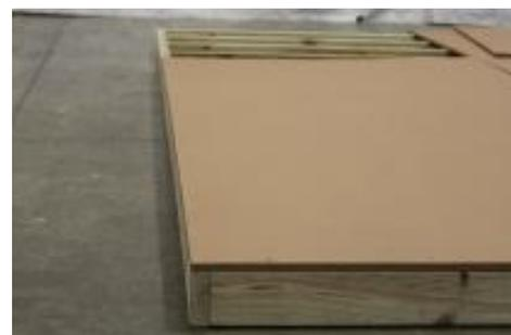
**(17)** Nail along the front side, making sure flooring is flush with the band board.
