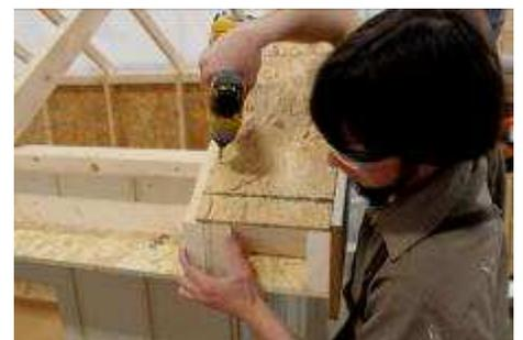
(106) Fasten gable overhang to rafter, using 2" screws, every 8 to 12 inches.
