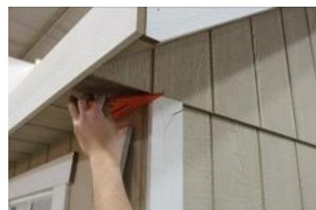
**(141)** Attach corner trim to gable wall, making sure it is flush with the front wall as shown, using 2" trim nails spaced 8-12" apart, along edge of trim.
