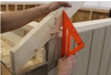
(95) Screw rafter to top plate, using a 3" screw, making sure rafter is flush with the wall siding. Repeat for opposite end of rafter.
