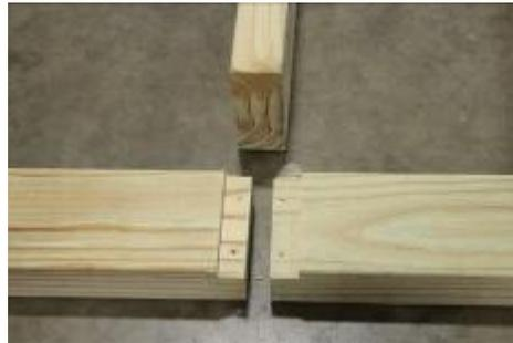
(5) **Note:** The band boards have dado grooves precut to ensure proper joist placement.
