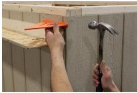
**(81)** Align siding flush with the top, and edge of front wall siding, using 2" siding nails.
