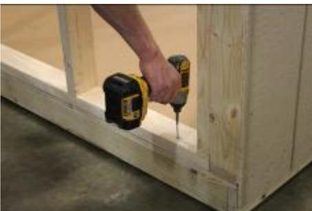
**(77)** Fasten to floor, using 3” screws, every 12 to 14 inches, trying to hit the floor joist.
