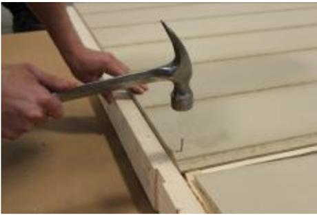
(35) Nail along the top, after making sure the siding is flush with the center of the double top plate as shown. Use an 8" to 12" nail spacing.
