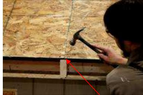
(120) Fasten the bottom left corner of the next piece of roof sheathing, making sure the edges are aligned perfectly.
