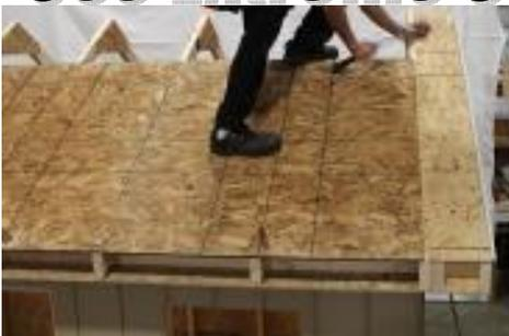
(122) Pull gable overhang parallel with the roof sheathing, then attach along gable rafter, using 2” nails every 8 to 12 inches.
