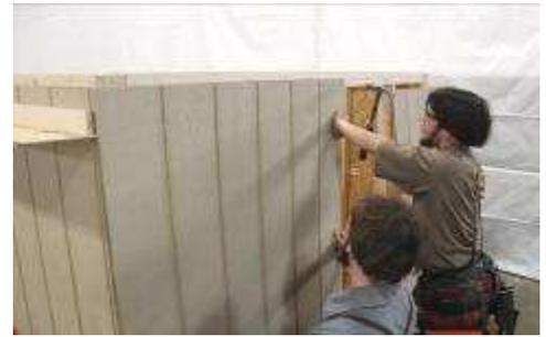
**(82)** Nail siding along top edge, making sure the siding is parallel with the center of the double top plate.
