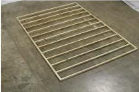
(4) After making sure the pad is level, locate the parts to assemble the floor joists, and scatter them out as shown.
