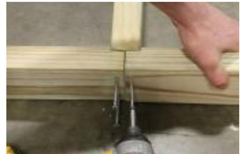
(9) Screw the rest of the band-boards into floor joists.
