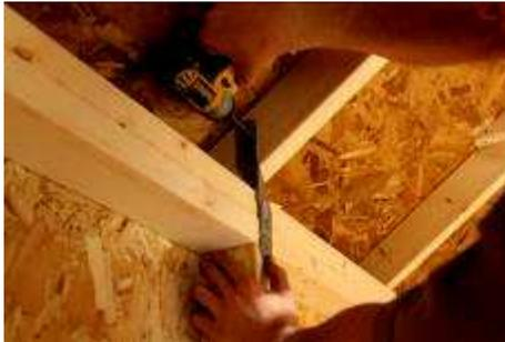
(164) Install hurricane ties, using 1-1/4" screws.
