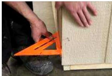
**(84) Correct!** Attach to wall studs, using 2" siding nails.
