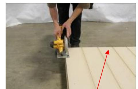
(43) Set the saw to 1/2" and cut along the line so that it is flush with wall frame. **IMPORTANT! Do not cut along the bottom of wall.**
