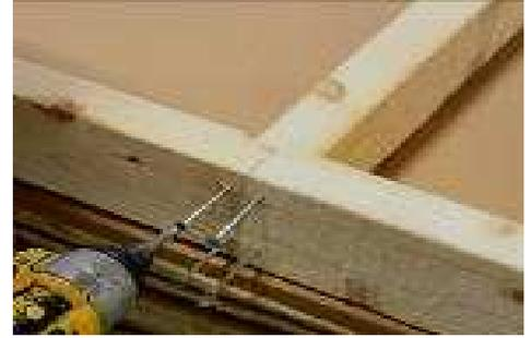
**(28)** Repeat the process for the rest of the wall studs; but use four 3” screws as shown, for any splice.
