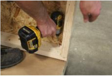
(53) Fasten to floor, using two 3” screws at every stud, trying to hit the floor joists.
