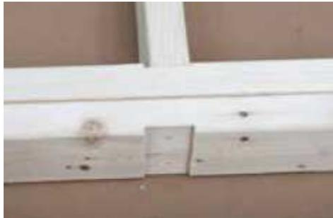
**(30)** Before fastening the double top wall plate, ensure that dado grooves align with wall studs, and are faced outward.
