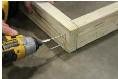
(8) Attach the band board, using 3" screws, through the pre-drilled holes.
