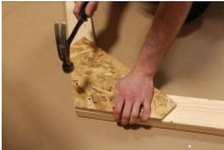
(92) Assemble each rafter by attaching one gusset to each side of the rafters as shown, using a total of ten 2" nails per gusset.
