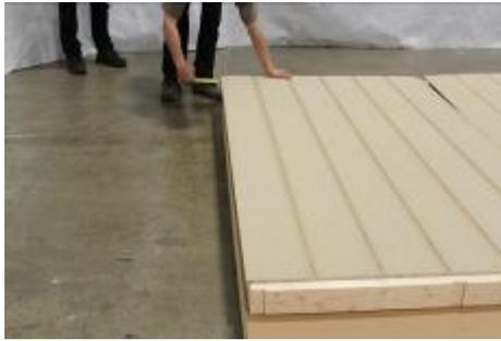
(36) Nail along the end, making sure siding is 1/2" out over the wall stud.
