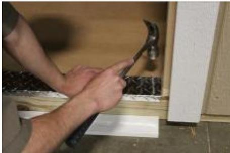
**(146)** Install diamond plate as shown, using two 2" nails every 10 to 12 inches.
