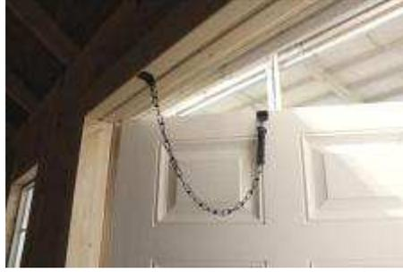
(162) Fasten the other section of the spring to the door, using two 1-1/4" black screws.
