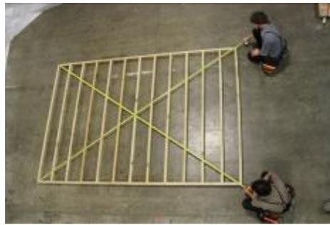
**(11)** Before proceeding, ensure that floor is square. Both measurements need to be equal.
