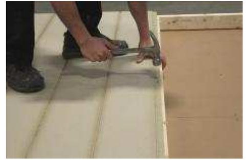
(37) Ensure that stud is parallel with siding, before nailing. Then firmly attach siding section along all edges and into each wall stud, using an 8" to 12" nail spacing.
