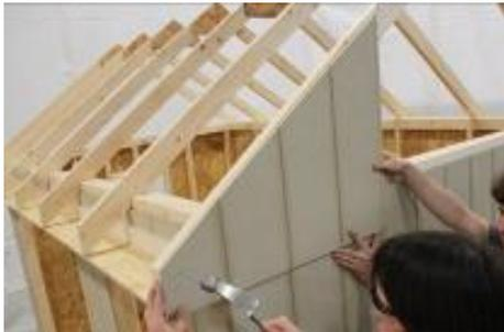
(101) Install the piece towards the front first, making sure it is aligned with the rafter and the chalk line.
