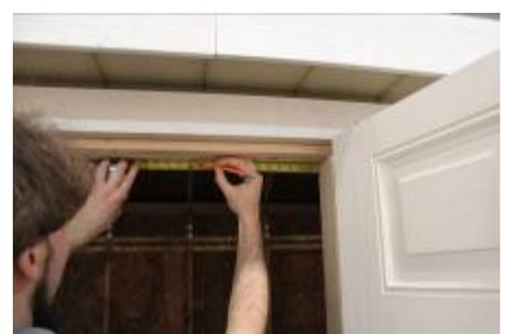
**(160)** Make a mark at 12", then install door spring, as shown in next step.
