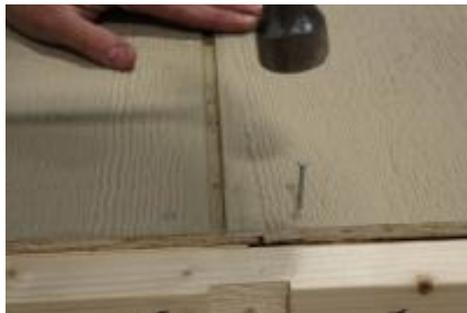
(38) Put the next piece in place, flush with the previous piece, making sure the splice looks similar to the other grooves. Then fasten the corner of the siding to the plate.
