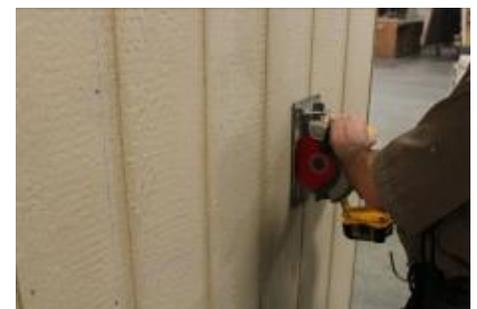
**(88) Remove the screws and chalk line,** then; set the saw at 1/2", and cut along the lines.
