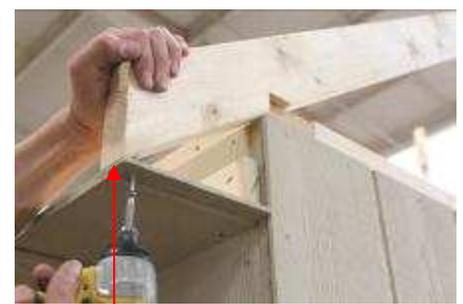
(94) Align rafter flush with edge of soffit, then screw soffit to rafter, using 3" screws. Repeat for opposite end of rafter.
