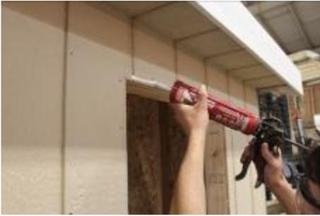
**(134)** Caulk around the perimeter of the window, and in every groove along the top, before moving to next step.
