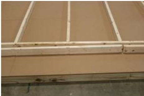
**(29)** Attach all wall studs to top and bottom and wall plate.
