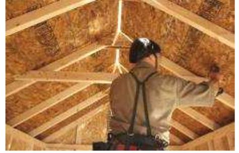
(163) Fasten the crosstie, using 3" screws. **Note: Divide the crosstie out equally.**
