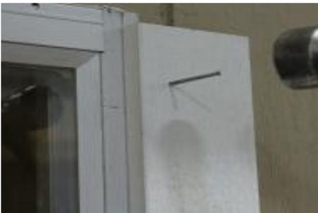
**(137)** Align side trim piece along the lines on the window frame as shown and attach using 2" trim nails. Repeat for the left trim piece.
