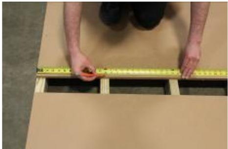
**(22)** Before you finish attaching the first row flooring to the joist, make marks 12" on center for a guide to adjust the joist when nailing.
