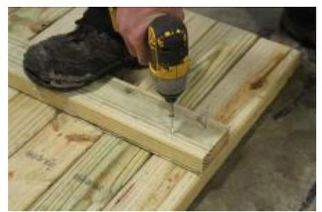
(169) Attach crosspieces to ramp boards, using two 2" screws per board. Countersink the screws approximately 1/4"
