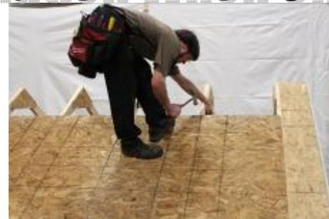
(123) Adjust the rafters to align with the marks you had made in step (126), then fasten the top of the roof sheathing to rafters. Finally, nail the rest of the roofing, using an 8 to 12 inch nail spacing.
