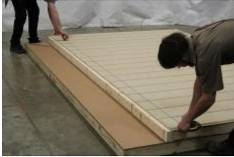
(45) Snap a line, using the marks from the previous step.
