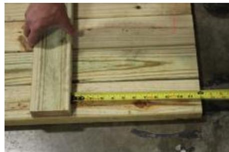
(168) Attach cross piece 12" up from end of ramp.
