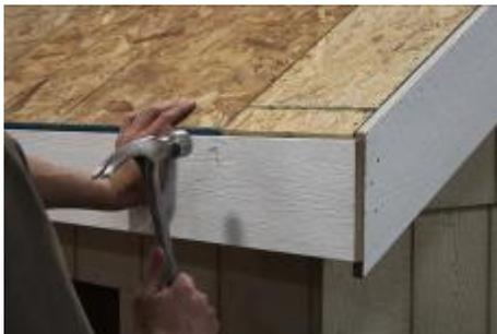
(128) Fasten to rafters, using two 2" trim nails per rafter, and making sure fascia is flush with the top of the rafters, and with the gable fascia.
