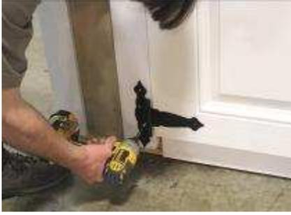
**(152)** Fasten the other hinges, keeping door flush with the trim on the left side.
