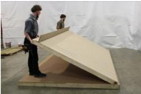
(50) Set the wall, making sure edges of wall are flush with edges of floor. **Note: It is VERY important that a person holds the wall in place until wall is attached firmly to floor, or braced.**
