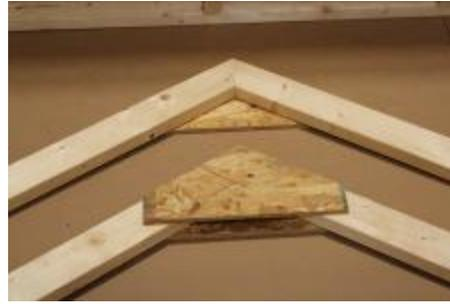
(90) Lay out the rafter pieces and the gussets. **Note:** Two rafters will be assembled using only one rafter gusset, the remaining rafters will be assembled using two rafter gussets.
