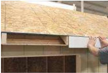
(126) Hold the fascia in place, making sure it is centered with the rafter, then move to next step before nailing.
