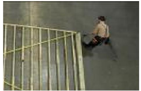
**(12)** Knock the joists on the end accordingly, till measurements are equal.
