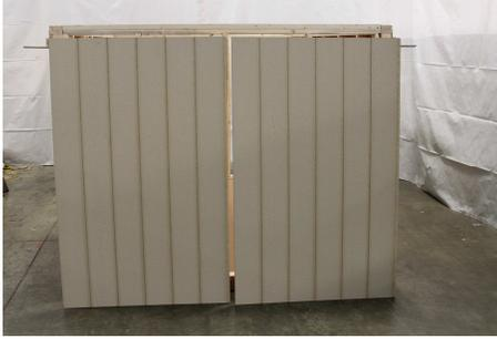
**(80)** Locate and lay out the gable siding with overlap towards the front.
