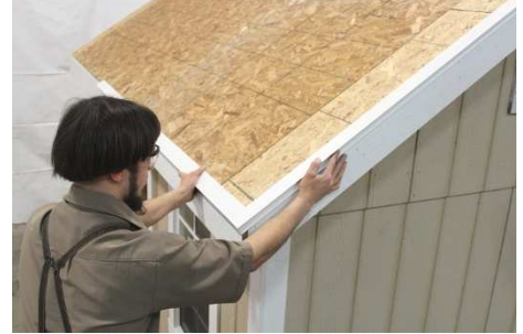
(172) Overlap the gable piece over the bottom piece and nail only the bottom.
