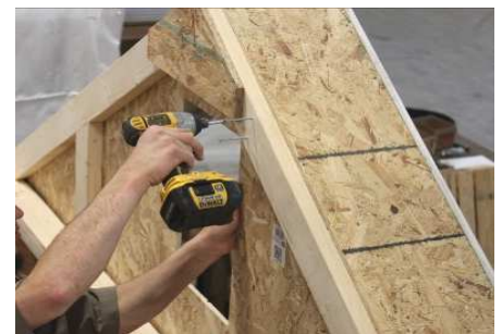
(112) Properly secure gable overhangs with 3" screws, every 10 to 12 inches.
