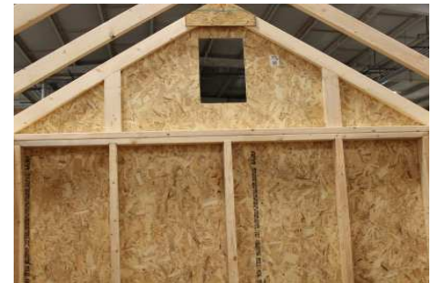
(115) Fasten the other gable brace on this gable, then repeat for opposite. Next, fasten the siding splices to the gable braces on the outside.
