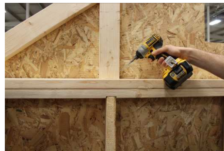
(114) Fasten the bottom of the gable brace on both sides.
