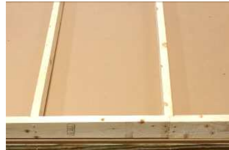
(75) Attach all wall studs to top and bottom wall plate.
