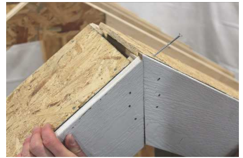
(109) Incorrect! Before fastening the overhangs on the top, make sure the splice is uniform, as shown in next step.
