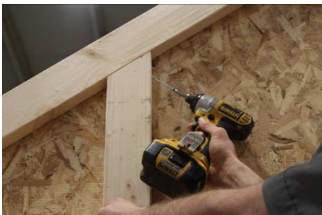
(113) Locate the 4 gable braces then fasten them at the siding splices in the peak, using 3" screws.
