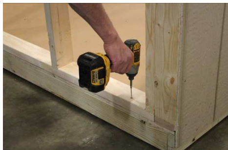
(78) Fasten to floor, using 3" screws, every 12 to 14 inches, trying to hit the floor joist.
