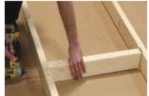
(76) Fasten the window blocks.
