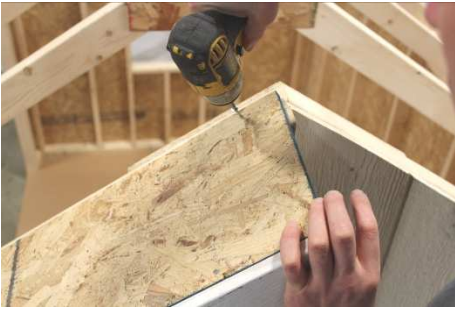
(107) Fasten the top as shown.
