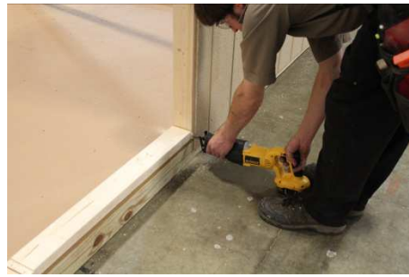
(72) Cut out bottom plate at door opening, using a sawzaw.
