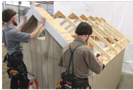
(108) Install right gable overhang, repeating previous steps.
