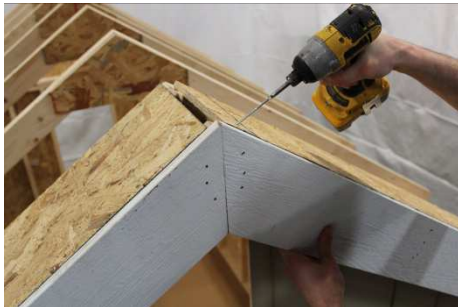
(110) Correct! Fasten firmly, using a 3" screw.
