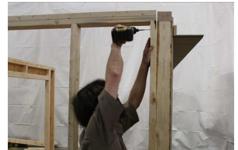
(79) Align gable wall framing flush with back wall framing and attach using 3" screws, every 8 to 12 inches. Repeat the process on opposite end.
