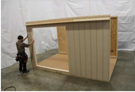
(71) Properly secure or brace the front wall, then move to next step.
