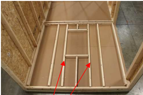
(74) Locate and lay out the parts to assemble the gable wall with a window. Note: Locate the window studs with dados, for the windows. Gable walls are interchangeable. Place window on desired gable wall.
